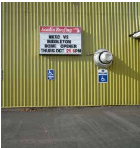
PA 5 | Accessible parking signage at Glooscap Arena
