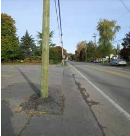
PS 1 | Uneven sidewalks in front of Port Williams Library
