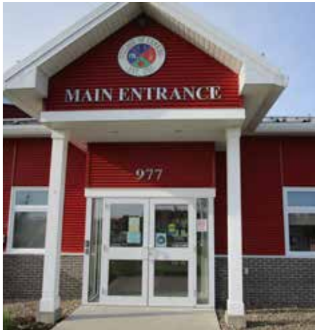
KA 7 | Front entrance to the Canning Fire Hall
