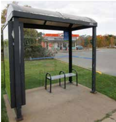
TR 3 | New Minas bus stop with accessible space next to bench
