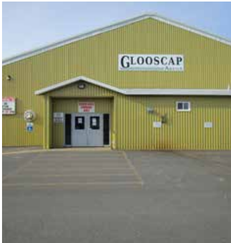
KA 4 | Front entrance to arena
