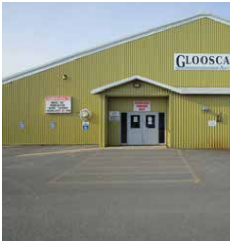
PA 4 | Accessible parking at Glooscap Arena
