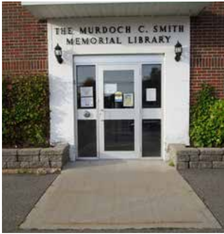
KA 2 | Accessible front entrance at the Memorial Library in Port Williams
