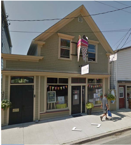
KA 1 | Front entrance to a building along main street in the Village of Canning
