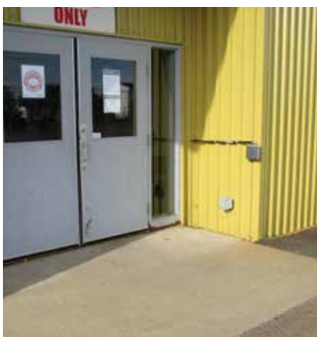
KA 6 | Power Door Control at Entrance
