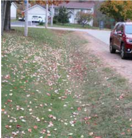
PS 3 | Lack of sidewalks forces users to walk along an active roadway
