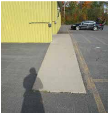
KA 5 | Accessible ramp to the south of the front entrance
