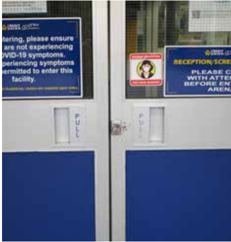
WS 1 | Credit Union Centre front entrance doors
