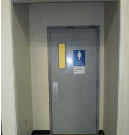
WS 4 | Womans washroom door at Glooscap Arena.
