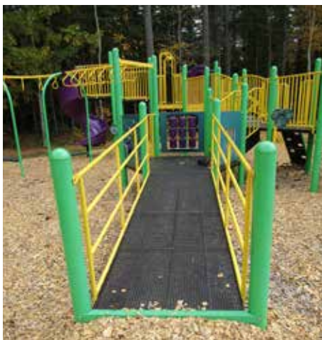
KA 15 | Ramp leading onto an accessible playground structure
